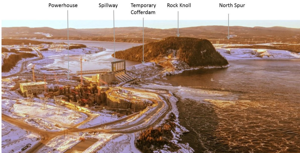
Figure 4.2. Muskrat Falls Hydro Facilities with the North Spur to the right, SNC Lavalin (2017). http://muskratfalls.nalcorenergy.com/wp-content/uploads/2017/01/North-Spur-Information-Session-Presentation__Jan-2017_Website-posting.pdf
