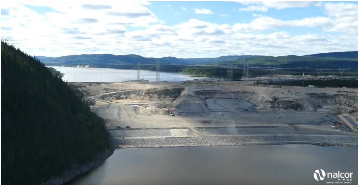
Figure 4.5. Stabilization of the downstream riverbank, August 2016, https://muskratfalls.nalcorenergy.com/newsroom/photo-video-gallery/muskrat-falls-construction-august-2016/
